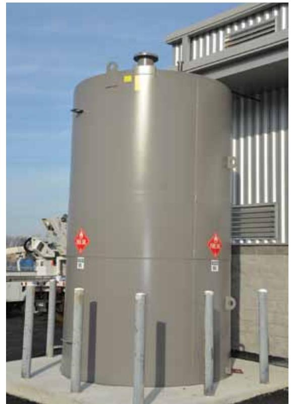
Used motor oil is pumped via a central collection system into a 5,000-gal. vertical holding tank, which then feeds two 375,000 Btu Energy Logic boilers.
