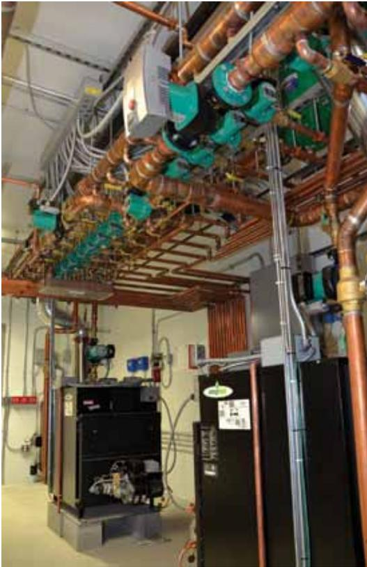
The Energy Logic boilers are backed up by three Baxi wall-hung 379,000 Btu condensing gas boilers. The design heat requirement is 1.2 million Btu of gas boilers, of which 750,000 Btu is offset by the waste oil boilers.
