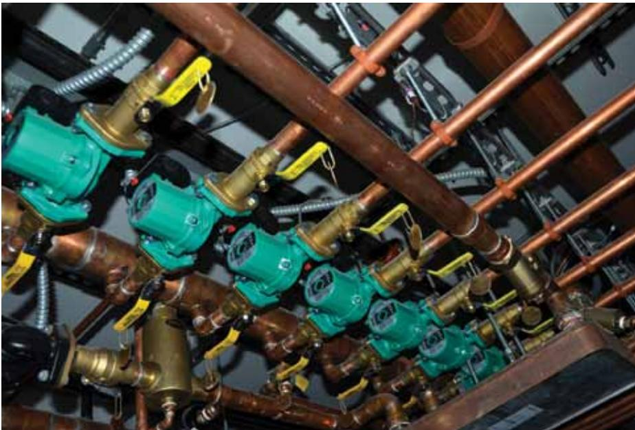
The mechanical system benefits from the use of Webstone Valves isolation flanges on the circulators, as well as Webstone air eliminators. The air eliminators significantly reduce installation and startup time by extracting air out of the system much more quickly.
