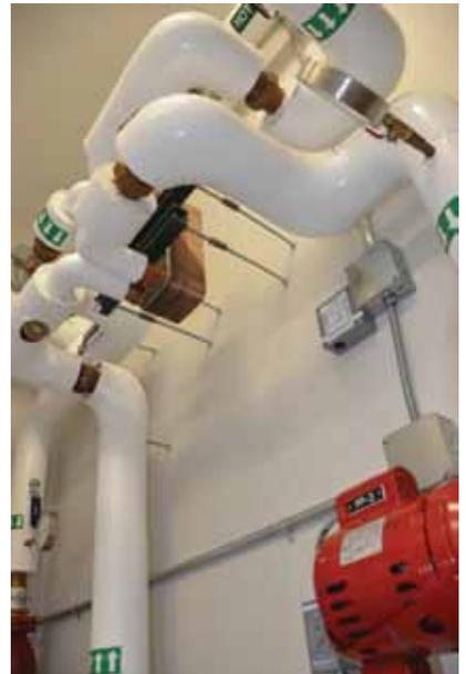
**A brazed-plate heat exchanger allows the pressurized and atmospheric portions of the system to work together seamlessly.**
