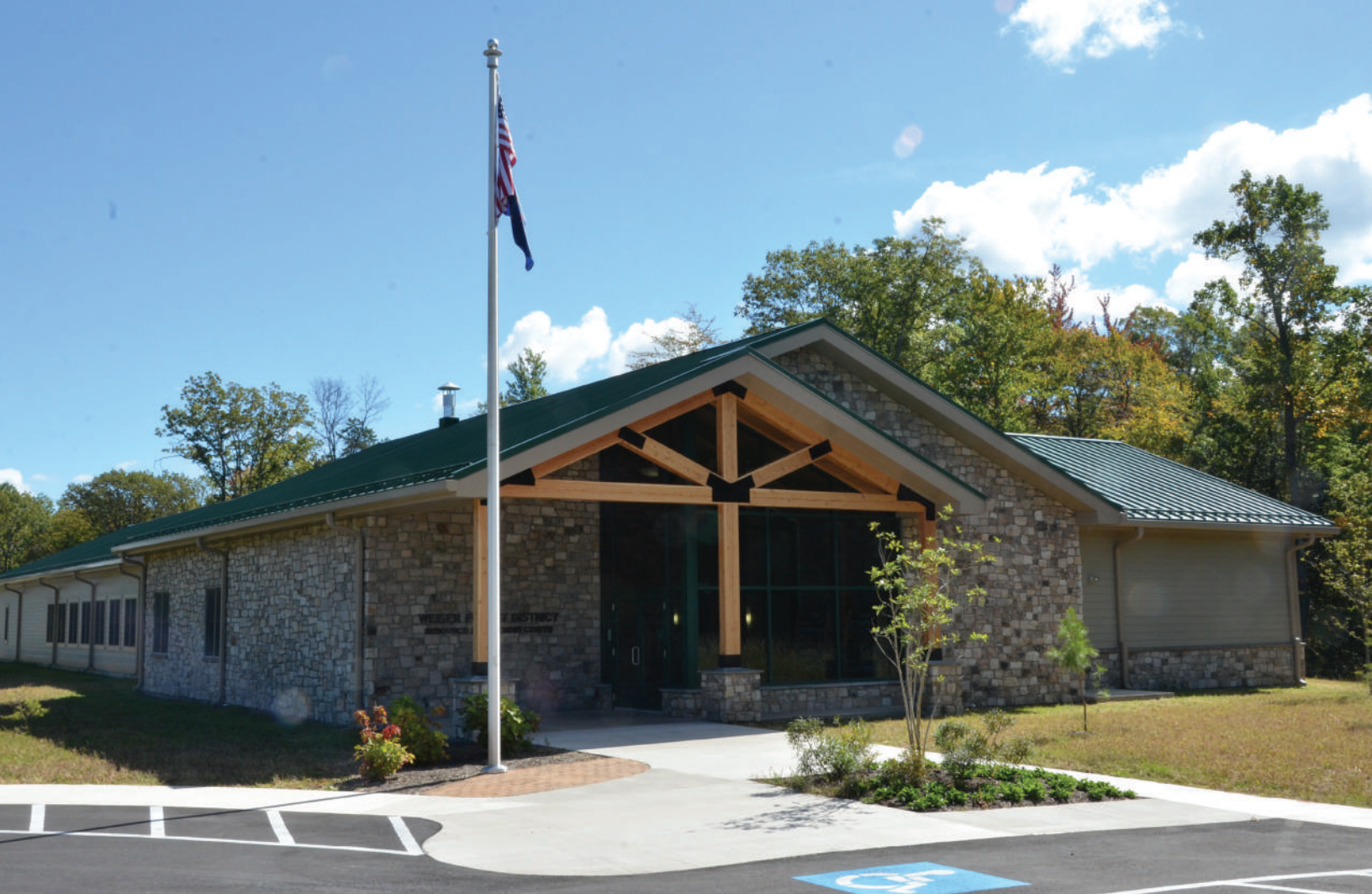
The new office building is heated via water pumped under the parking lot from the main mechanical room.
