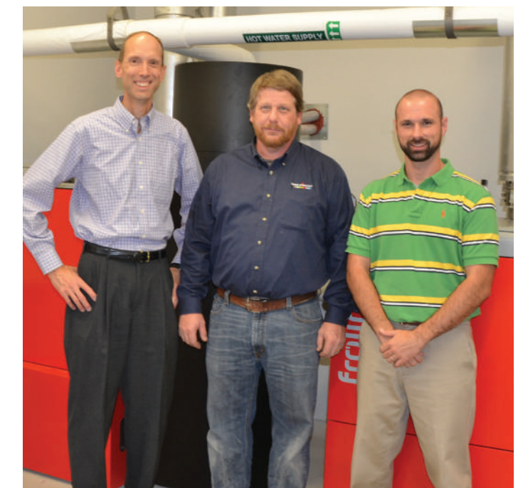
(L-R) Carl Longenecker, owner of ATI Systems, René Ferland, sales & technical support for Tarm USA, and Jason Adams, C.B.C.P Mechanical Engineer II, with Pennsylvania DCNR, stand in front of the two pellet boilers.
