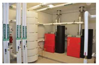
The boilers operate at near-condensing efficiencies. Everything from ignition to pellet loading is automated. The boilers share a main mechanical room with a superinsulated, 400-gal. buffer tank. All supply and return lines run underground.
