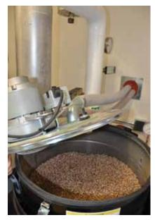
The wood pellets, seen here inside of a day bin, are sawmilling byproducts. Only compressed wood—no bonding agent—is used in the making of the pellets.
